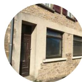
LA MAJORITÉ DES BÂTIMENTS ANCIENS ONT ÉTÉ CONSTRUITS AVEC DES MATÉRIAUX LOCAUX, PRINCIPALEMENT DU CALCAIRE. LE CHOIX D'ENDUIRE OU NON LA FAÇADE DÉPEND DE PLUSIEURS FACTEURS, NOTAMMENT LA NATURE ET LA RÉSISTANCE DE LA PIERRE, LA QUALITÉ DE LA MISE EN ŒUVRE DES MOELLONS ET LA STRUCTURE DU BÂTIMENT.
